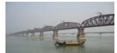
Hardinge bridge across the Padma (Ganges)
