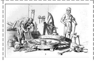
You are a wheelwright. Your apprentice carves the spokes with a two handled knife. You fix the spokes on the axle and then put on the rims. These are in three or four parts. You then have to roll the wheel to one side to wait for the smith. He or she has to fix the iron ring round the rim.
