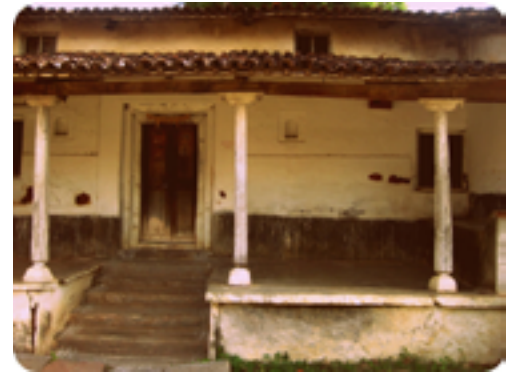
pyol: raised porch
