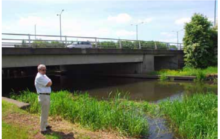
M4 motorway bridge over the River Colne © RGS-IBG Discovering Britain
